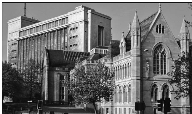
Figure 3. The magnificent Arkwright Building (1), with the Newton Building (4) beyond, both faced with limestones.
