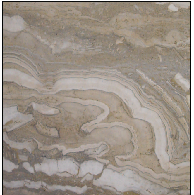
Figure 17. Travertine cladding on MacDonalds (83).
