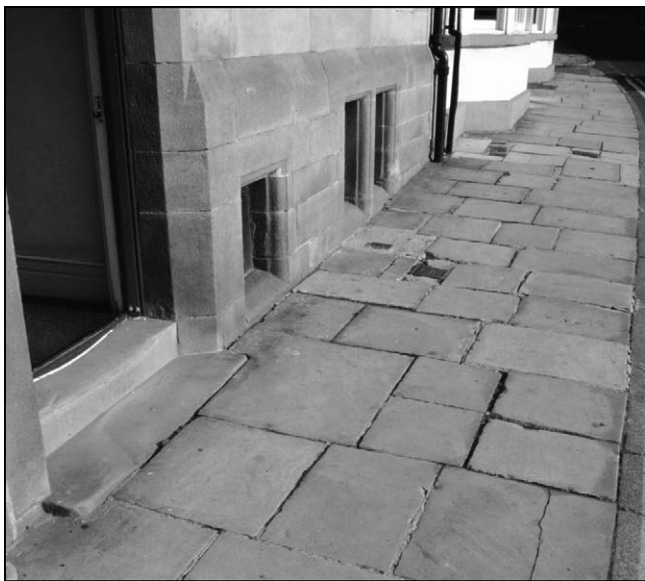
Figure 19. Flagstone paving on High Pavement (69).
