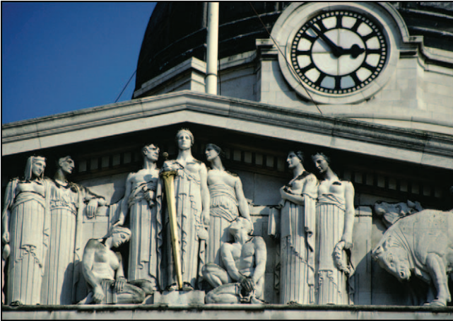
Figure 6. Portland Stone on the Council House (23).
