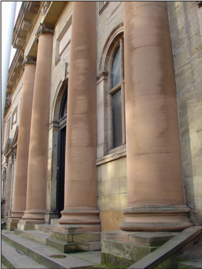
Figure 14. Sandstone frontage on Galleries of Justice (71).
